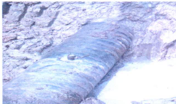
SPILL POINT AFTER EXCAVATION
