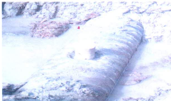
REPAIR WORK DONE BY NAOC REPAIR TEAM
