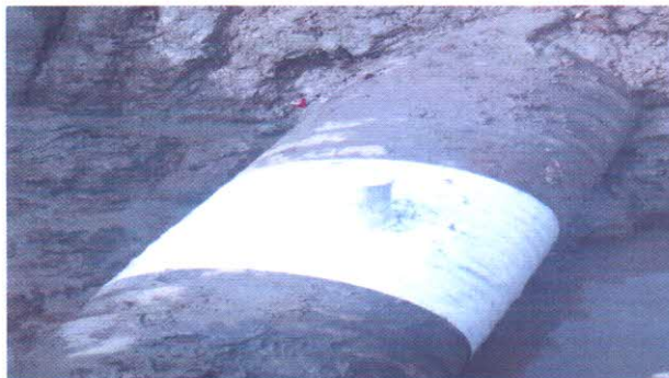
TAPE RAPPING OF SPILL POINT
